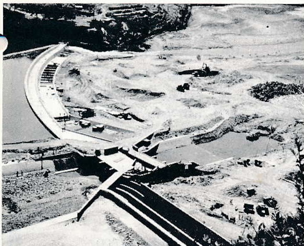
Jhimruk Hydro Power Project Dam Site, March 1993
